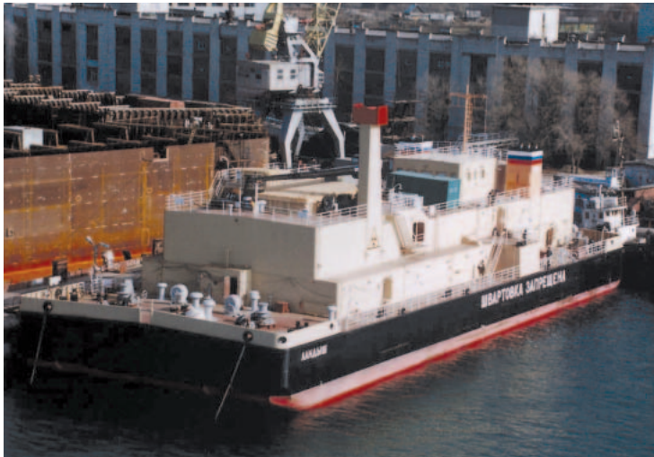
Photo: The liquid radioactive waste treatment facility “SUZURAN” constructed with the assistance of Japan
