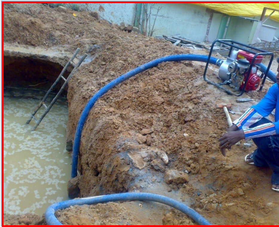
Plate 2.2 Water being dewatered from an open sump
