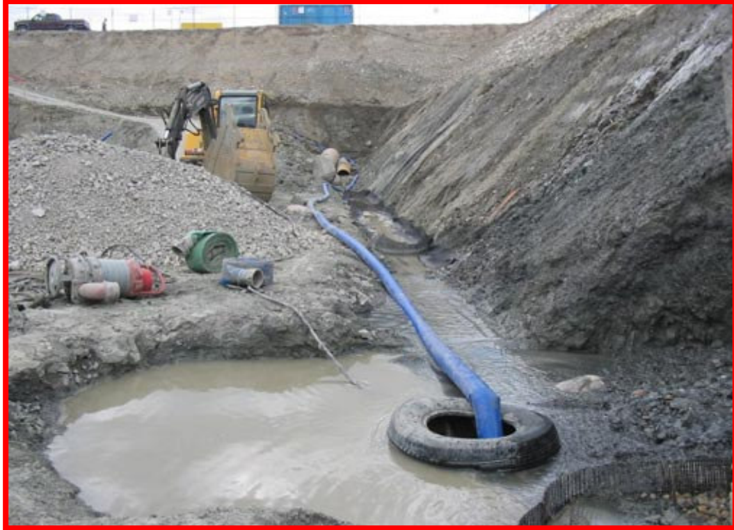
Plate 2.1 Water being dewatered from a ditch
