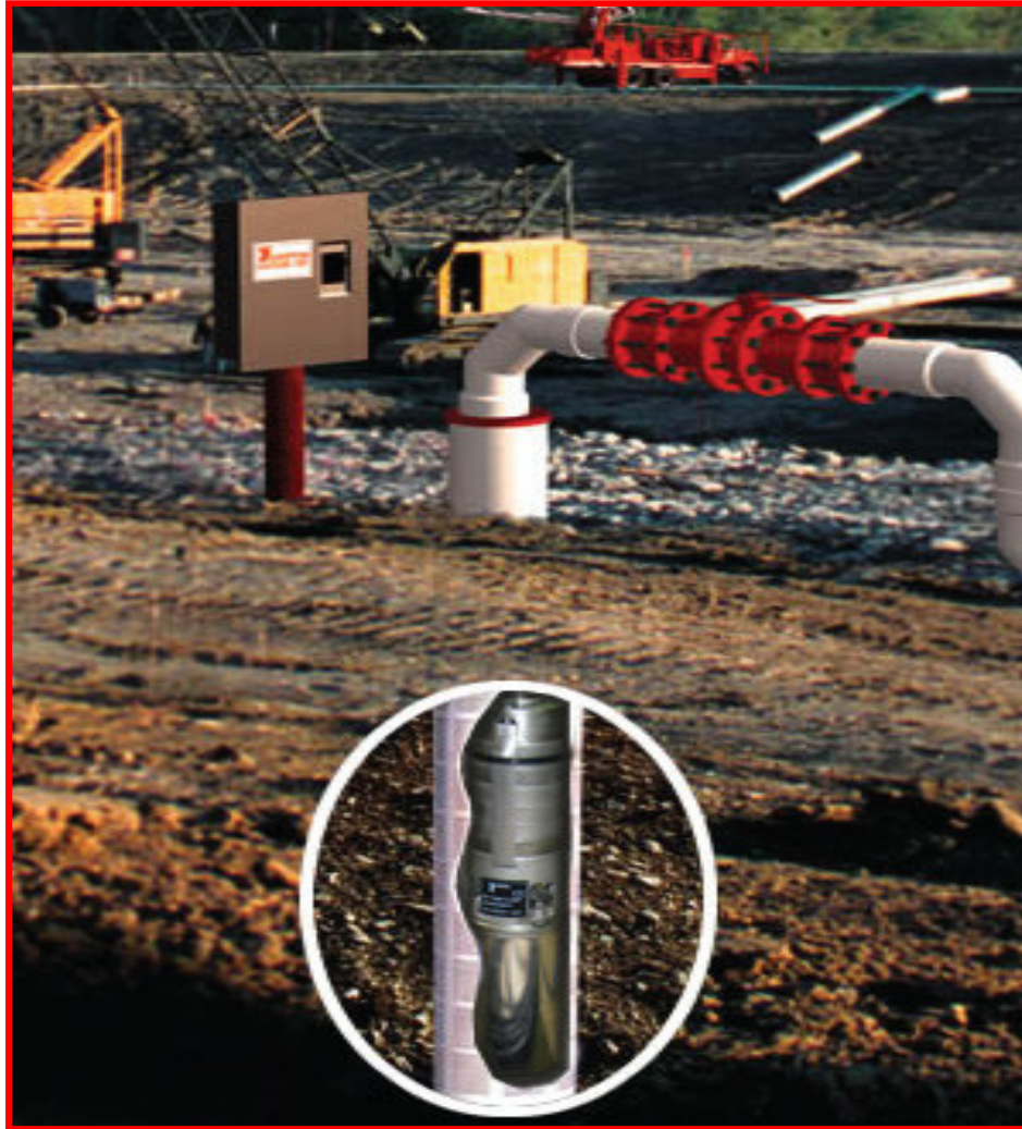
Plate 2.5 Installed deep well point
