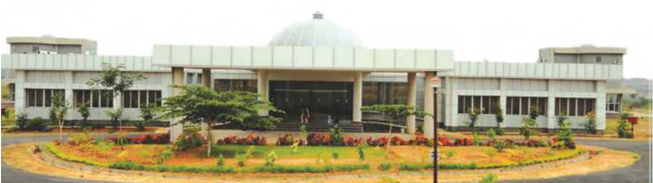
ISRO Navigation Centre (NIC) at Byalalu, the nerve centre of IRNSS Ground Segment
