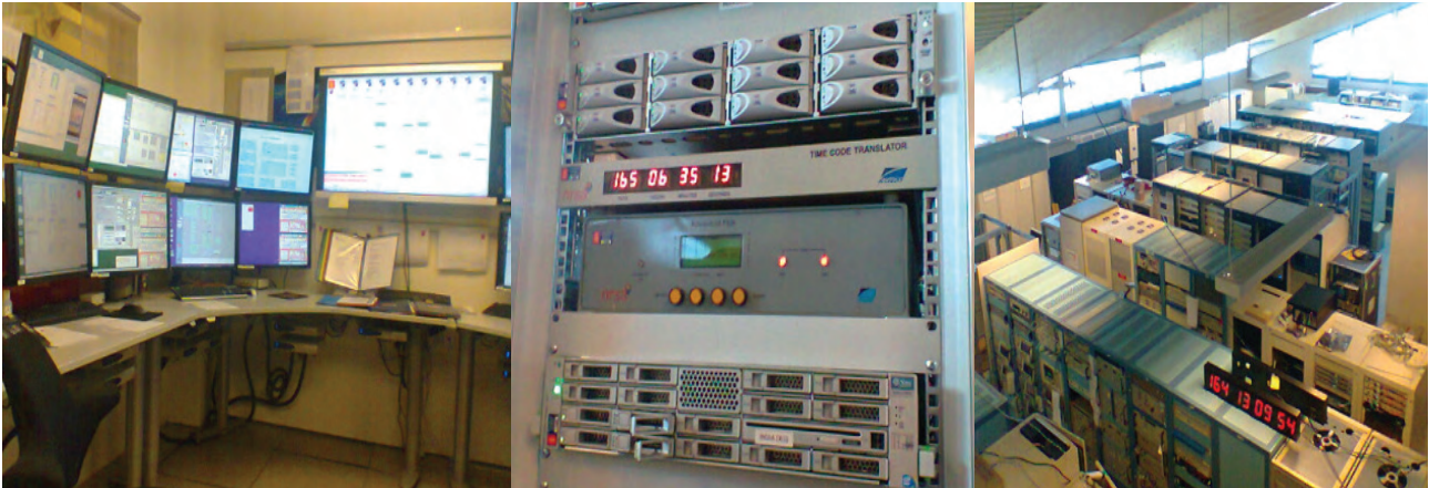
KSAT Data Reception Station Facility
