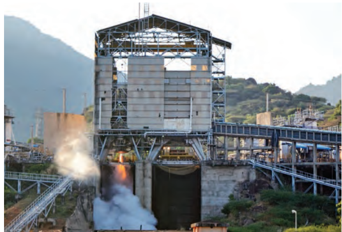
CE20 Engine Hot test
