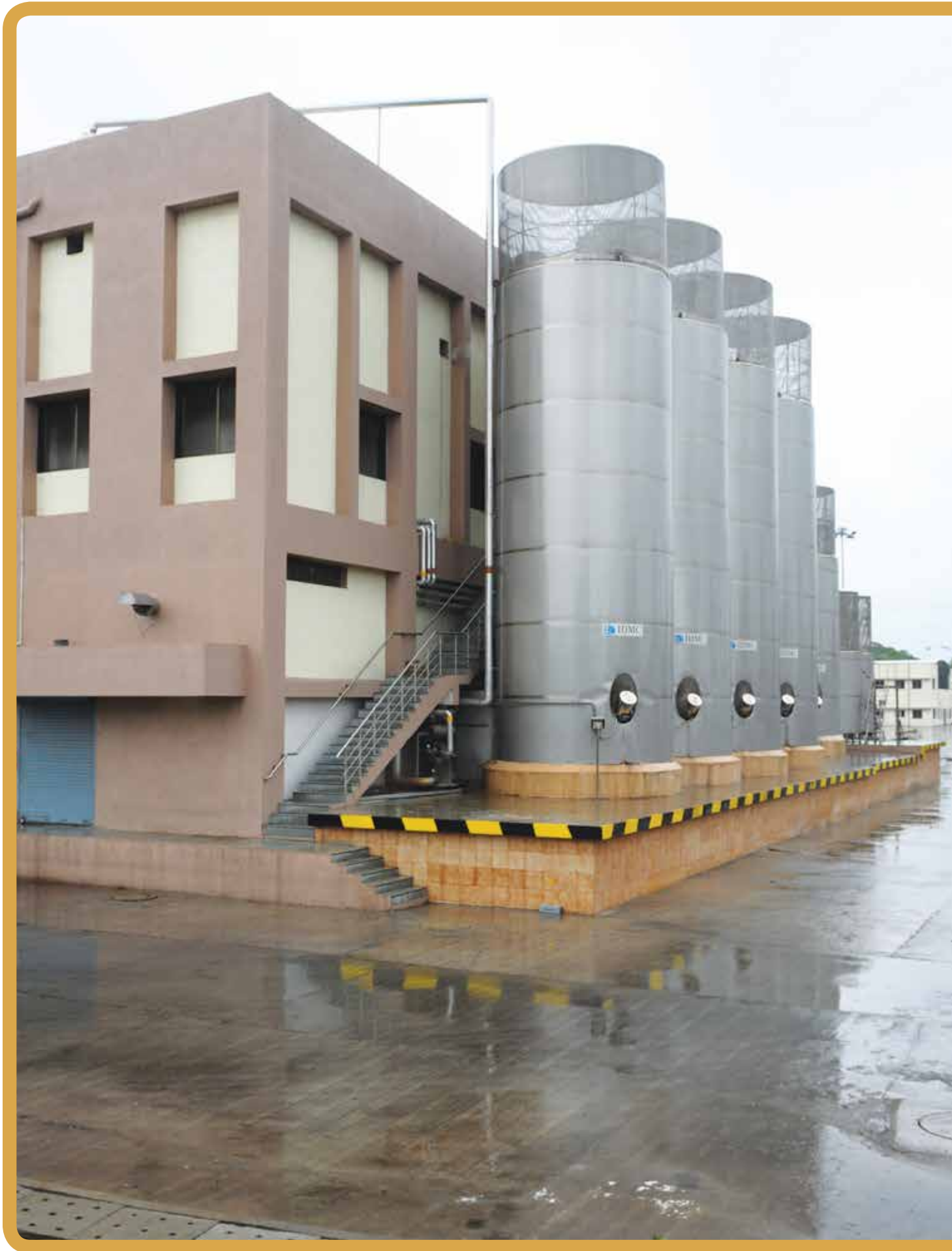
Dairy plant expansion, Rajkot
